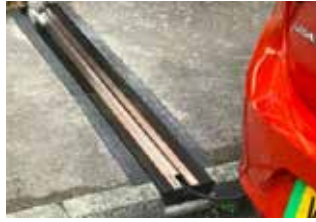
A pavement gully
